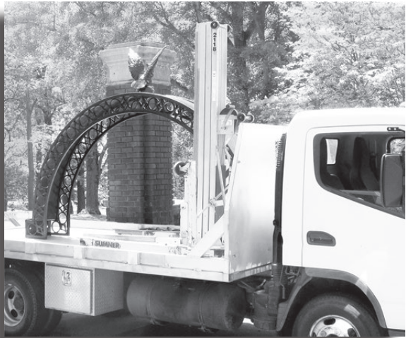
To the left, the southern arch rests on the bed of a truck, awaiting its reinstallation atop the brick columns.
