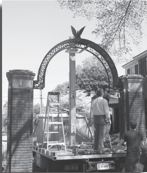
Below, the northern arch is held in place by the mechanical lift, in the process of being reattached to its columns.
