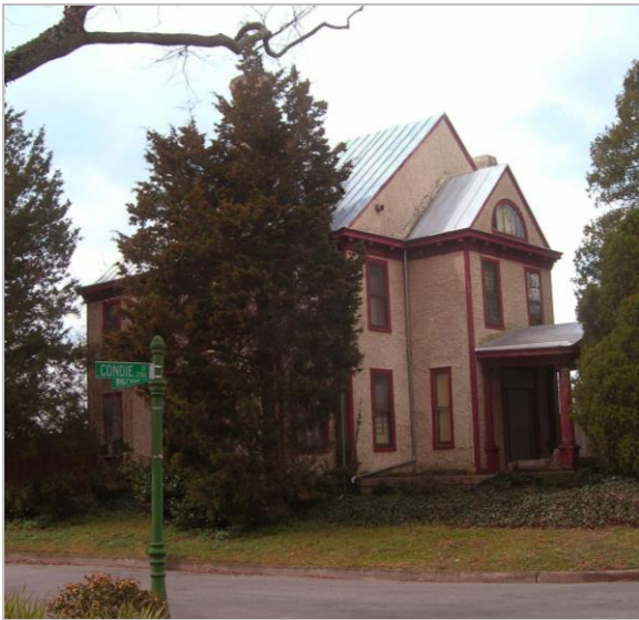
Fig. 7. Summer residence of Judge E.C. Minor, built ca. 1892. It stands today at the corner of Walpole and Condie Streets.
