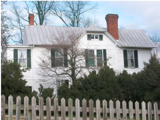
Fig. 9. Charles Euker built his “Marburg” residence ca. 1889-90 (view from the south). It presently stands at the corner of Bute Lane and Rugby Road but awaits impending demolition by its present owner/developer.
