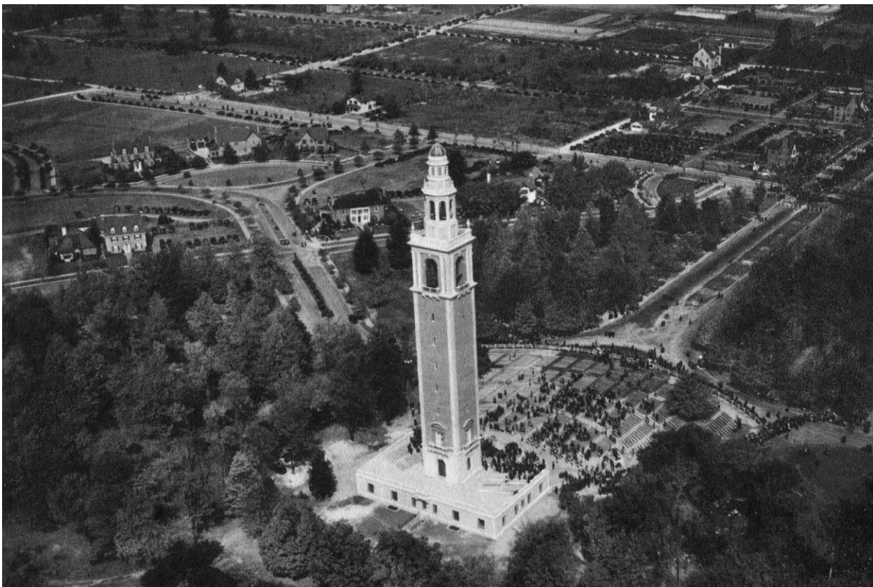
Fig. 21. Aerial view of the War Memorial Carillon dedication, October 15, 1932. Cadet regiments march down Blanton Avenue, here just arriving at Douglasdale Road. William Byrd Parkway development in the background. Courtesy, Dementi Studios.
