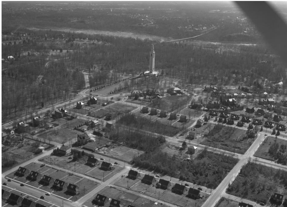
Figs. 23 & 24. Aerial views of new development west of the open-air reservoir, early 1950s. Top: The Rueger mansion has been demolished to make room for future John B. Cary Elementary School. Bottom: Looking toward the Carillon, the vista also includes new houses on Granite (later Garrett) Street and Grantland Drive. Courtesy, Adolph B. Rice Studio Collection, Library of Virginia.
